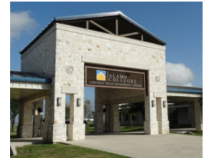
Central Texas Technology Center CTTC
